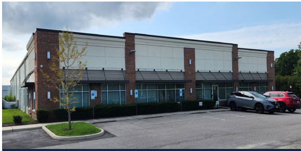
20,000 SF – Landscape Supply, LLC Virginia Beach, VA
