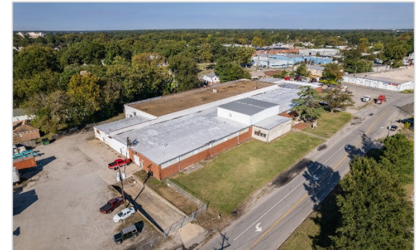
14,662 SF – A & J Trucking Repair, LLC Portsmouth, VA
