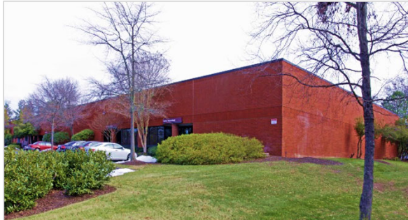
10,000 SF - Commonwealth Rest. Spec. Richmond, VA
